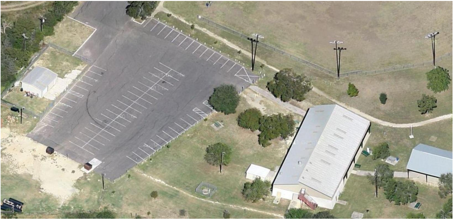
Aerial photo of facilities
